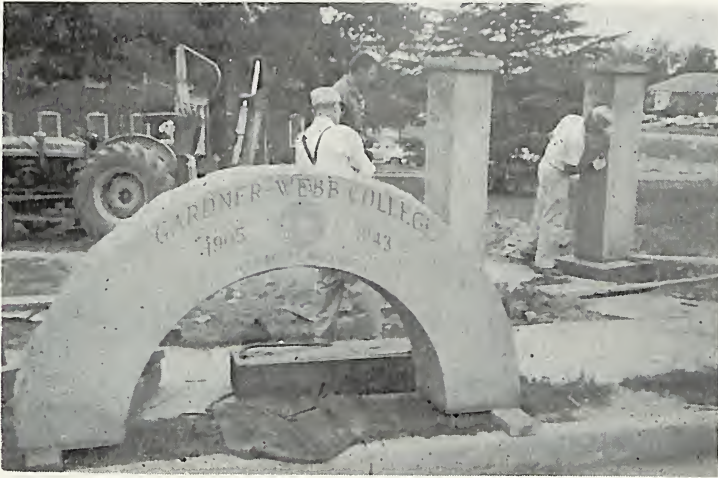
Workmen Are Shown Erecting Arch On New Location
